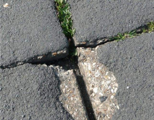
The poor condition of Tormead Road continues to deteriorate. The tarmac surface is worn out in many places by speeding cars, high tonnage vehicles, the bus service using this road and by school buses. The worsening road surface has exposed the concrete slabs which now show wear and tear particularly at the edges of the concrete slabs and where the road has been dug up through the concrete to access and service the major gas pipeline that runs under Tormead Road.
